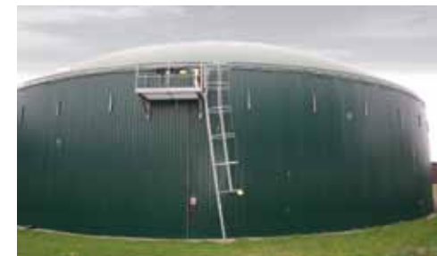
One of the three digester tanks
