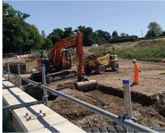
Excavation of the eastern swale, as part of the drainage works, near the connection at Barkham Brook
