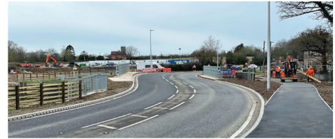
Barkham Bridge open to traffic
