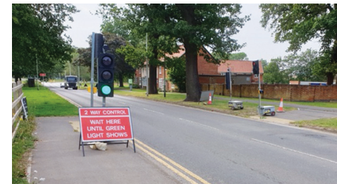
The temporary pedestrian crossing on Biggs Lane
